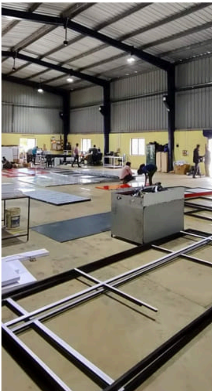
FABRICATION • FRAMES LAID OUT
