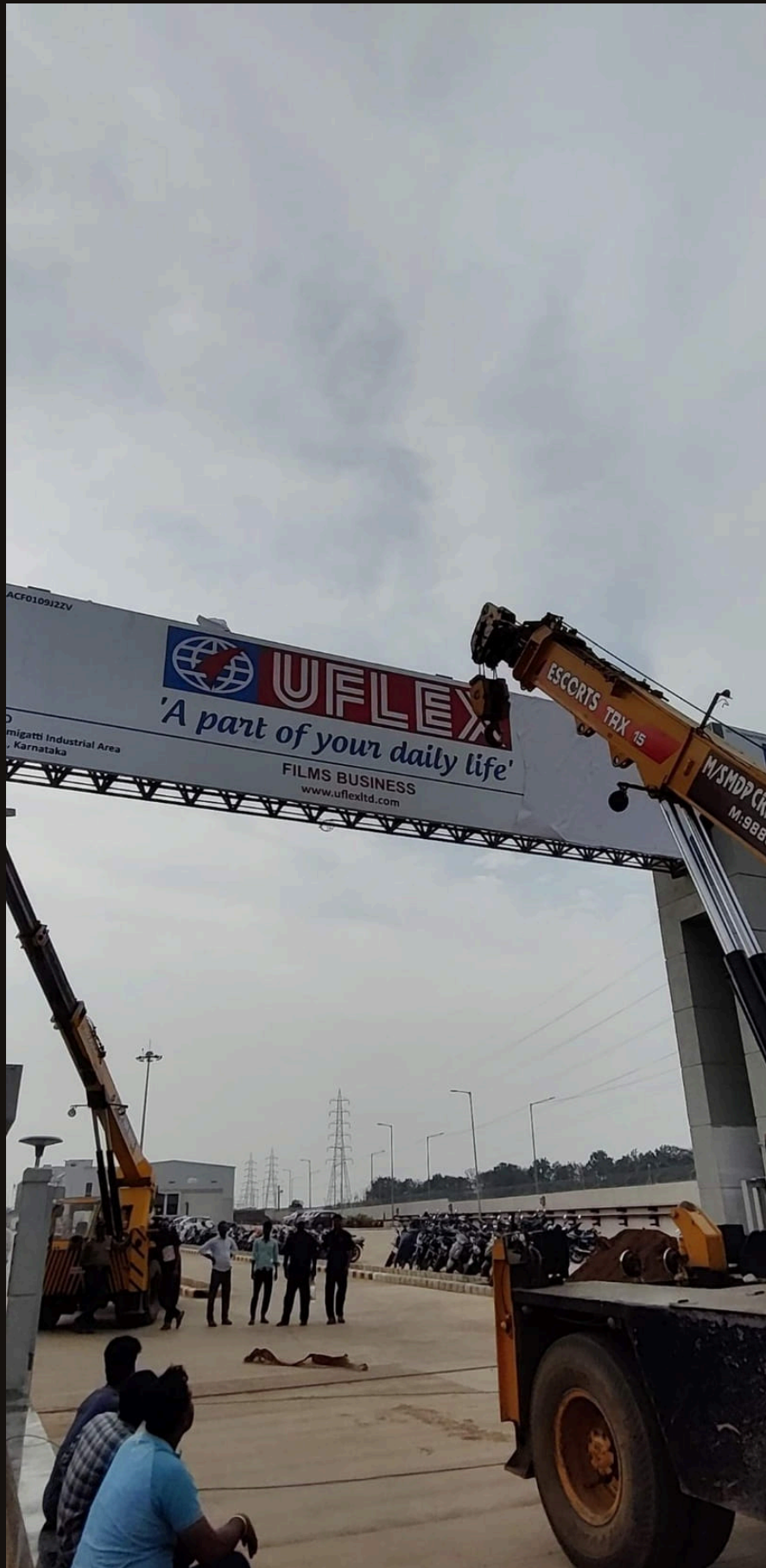
CRANE DAY • OVERHEAD GANTRY GOING UP
