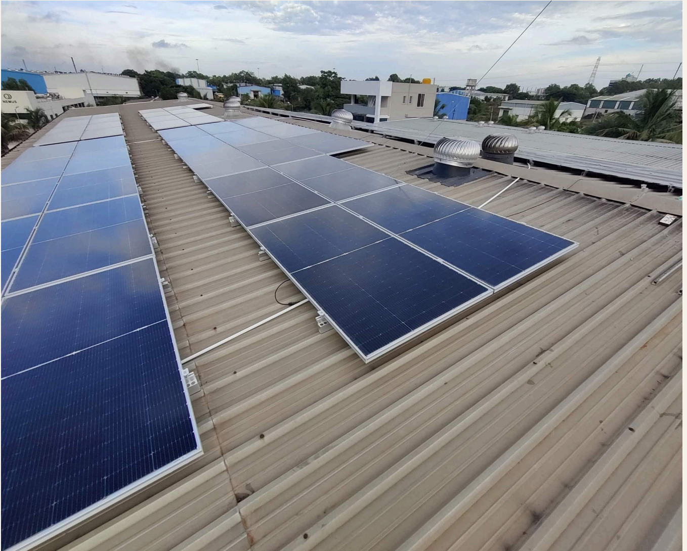
SOLAR • DAYLIGHT ON THE SHED ROOF
