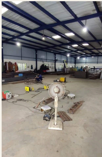
STEEL FRAME • BEFORE FIT-OUT
